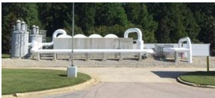
Fig 1. Horizontal biofilter installed in a concrete rectangular construction. Picture represented for illustration purposes only.
